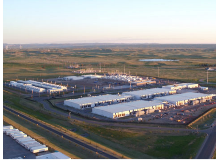
One of Microsoft's hundreds of data centres spread around the world where huge banks of servers power their company – including AI technologies – and it all takes vast quantities of water to cool.
