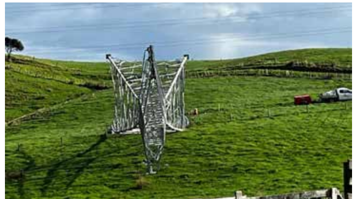
Maintenance crews undo all the bolts holding down a Northland power pylon and the predictable ensues – cutting power to much of the far north for several days in June.
